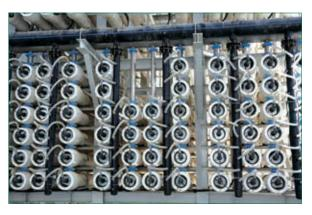
With five gas turbines and two steam turbines, the contracted power capacity of the Plant is 445 megawatts. The Plant's water production is based on a reverse osmosis process and the contracted water production capacity is 15 MiGD. The Plant entered into full commercial operation on 25 May 2012.
